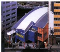
self-cleaning TiO 2 layer on a roof
